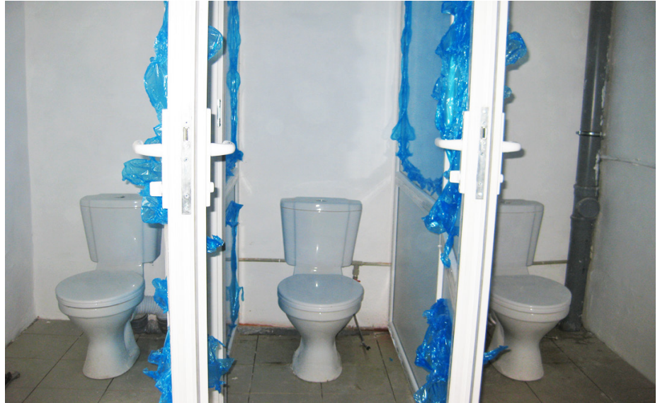
Renovated toilets in a dormitory in Yasynuvata
