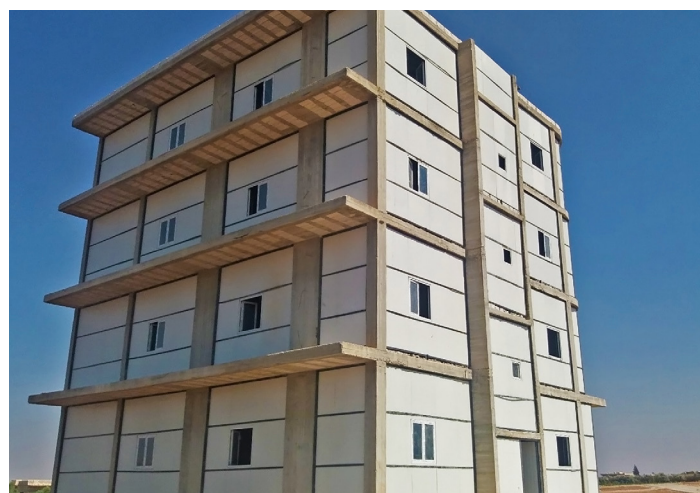
Unused building, newly refurbished by IOM and ready to house IDP families in northern Syria.
