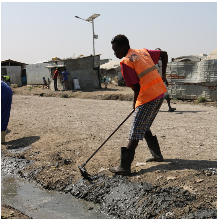
Drainage maintenance undertaken in Malakal PoC site. ©IOM/ Mominee 2018
