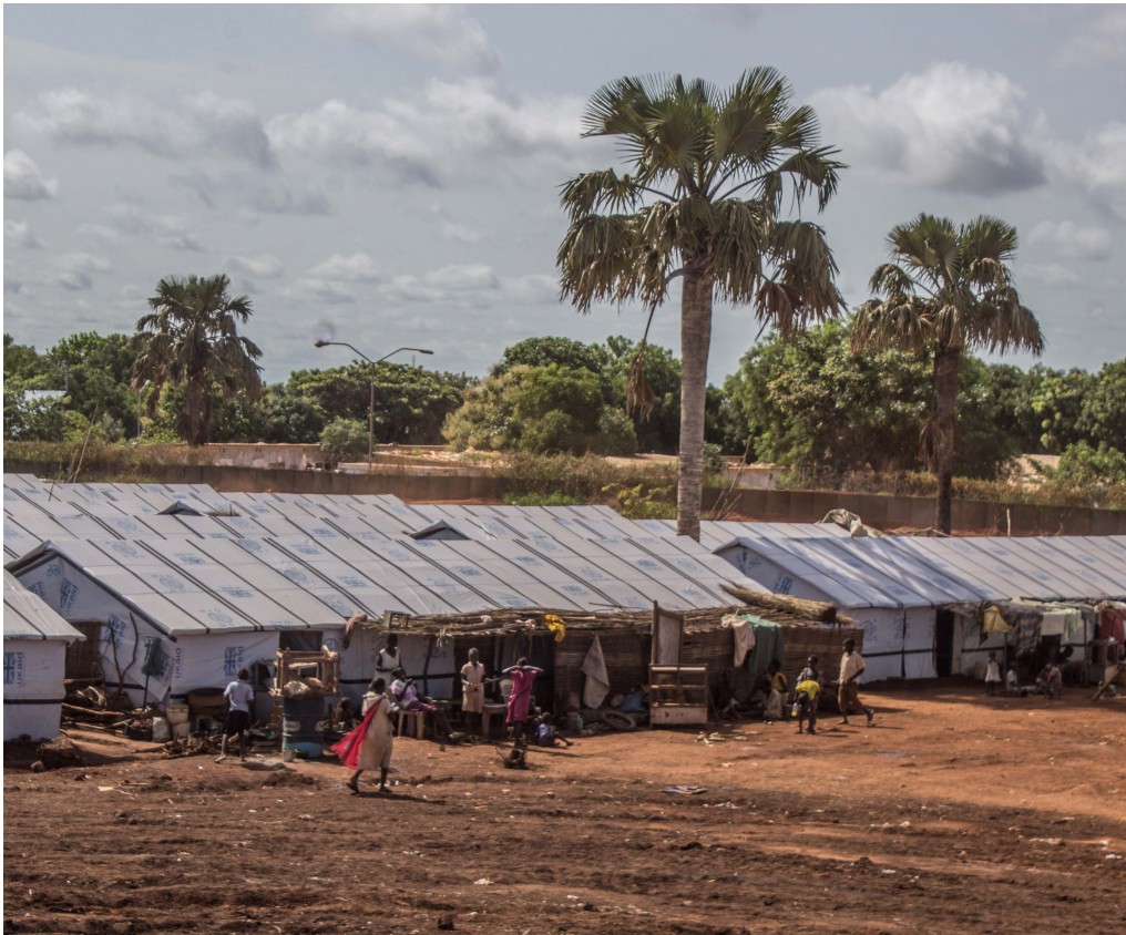
Newly rehabilitated area of zone A at the Wau PoC site. IOM/McLaughlin 2017
