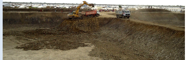
IOM work on the retention basin continues despite the rain
