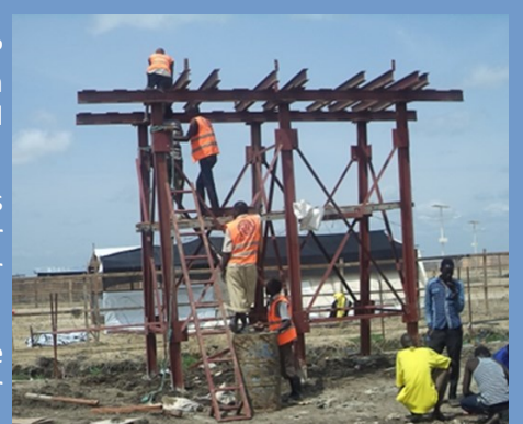
IOM constructs a water tower in the Malakal PoC extension site
