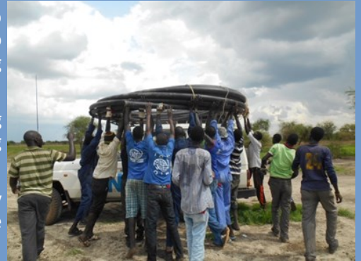
IOM installs pipes for water treatment plant in Malakal PoC
