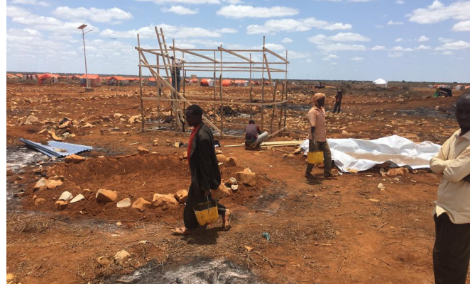
Construction of the health centre in Barwaqo 2 © IOM Somalia 2019
