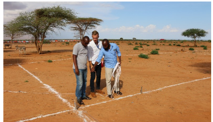
IOM staff and contractors surveying the expansion of the Kabasa internally displaced persons site in Doolow © IOM 2017
