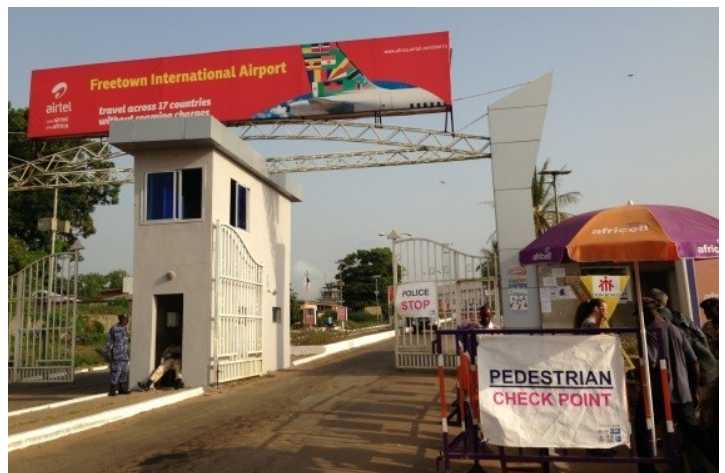
Lungi International Airport Front Gate and Inspection team © IOM 2015
