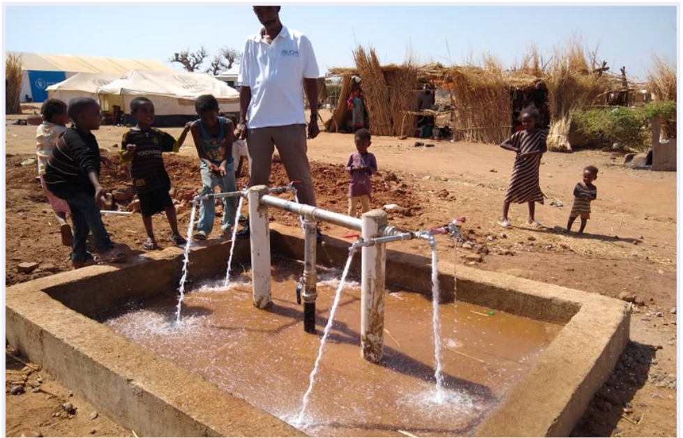
The newly completed, IOM-constructed water supply system in Um Rakuba Camp, Sudan © IOM 2021
