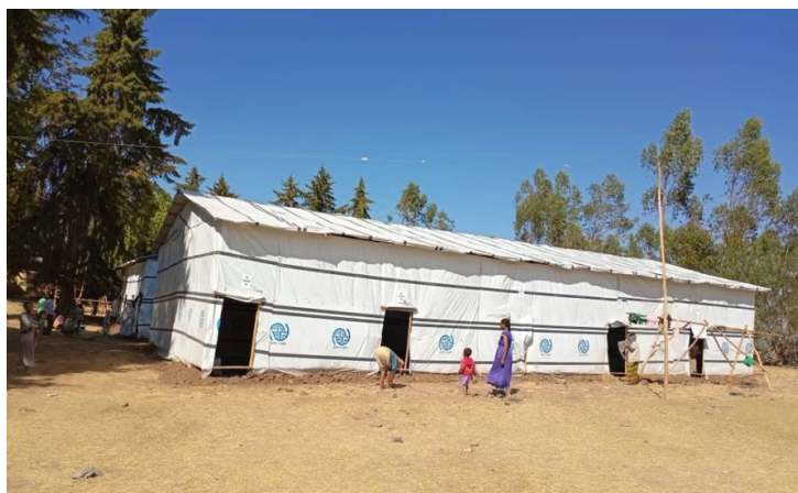
A communal shelter built by IOM in Dabat/Golmasa IDP site, Ethiopia © IOM 2020
