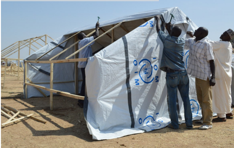
IOM shelter construction in Pulka. (Photo: © IOM/ Julia Burpee, 2016)
