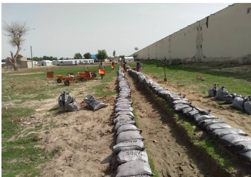
Local drainage construction at Stadium camp, Maiduguri © IOM 2019
