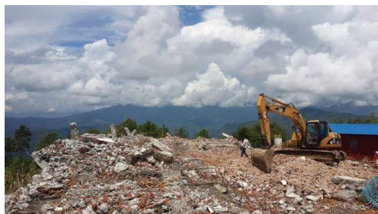
Shree Setidevi Higher Secondary School before and after demolition works (© IOM 2015 )
