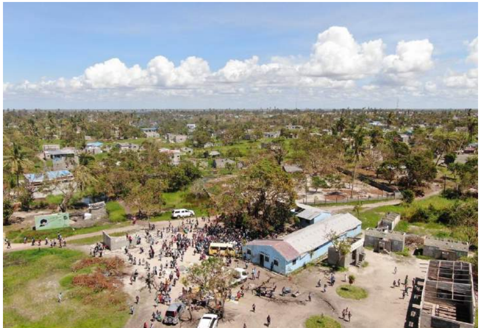
Tarps received from USAID where deployed by IOM to repair the roof of the Matadouro school building in order to allow classes to resume at the request of government authorities. © IOM 2019/P. Ocana
