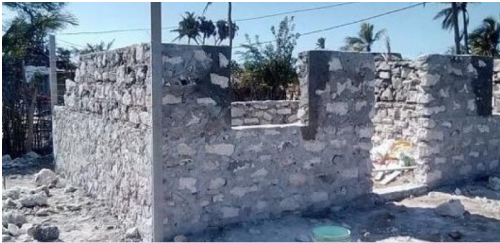
A house in Ibo Island, using structural walls technology, under construction through IOM implementing partner Instituto Oikos. © Instituto Oikos 2019
