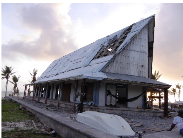
USAID plastic sheeting is used to cover Asor Men's House in Yap, FSM © IOM Micronesia 2015
