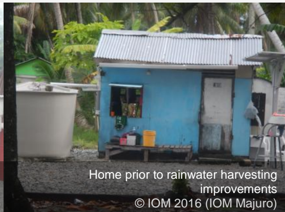
Improvements in progress © IOM 2016 (IOM Majuro)
