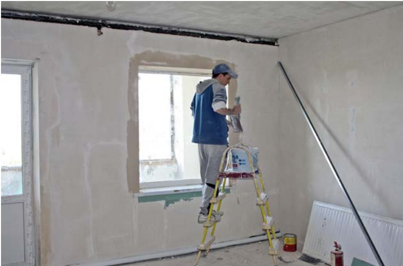
Renovation works ongoing. IOM supported the IDP community with construction materials
