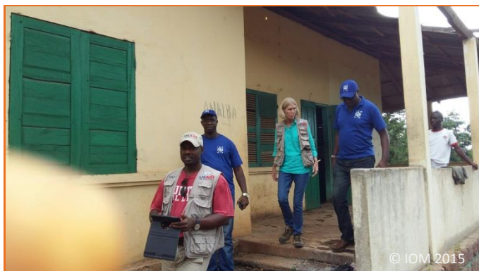
IOM/OFDA teams carrying out an assessment of the PEOC building before Rehabilitation-BOKE
