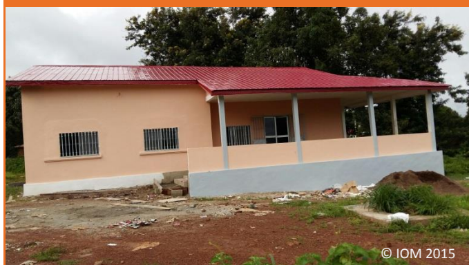
PEOC after Rehabilitation-BOKE
