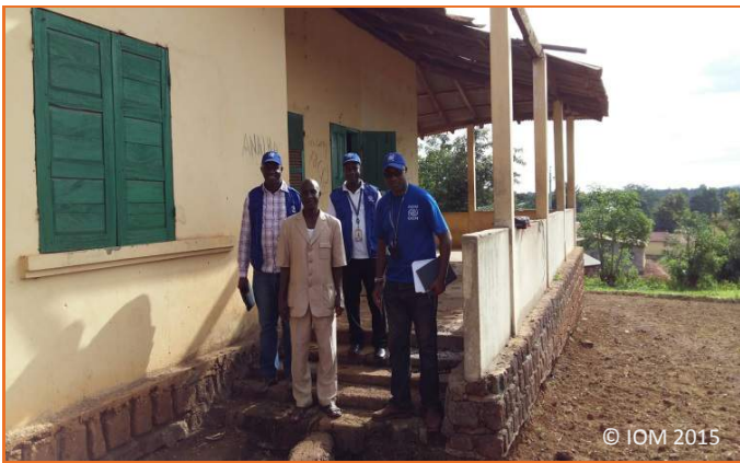
Building to be rehabilitated as PEOC in Boké
