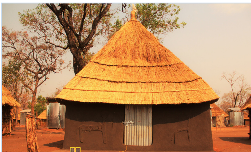
Transitional Shelter constructed by IOM with assistance from refugees in Jewi camp. Photo IOM 2017.
