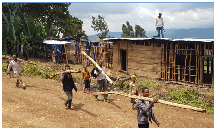
DISPLACED INDIVIDUALS CONSTRUCT TEMPORARY SHELTERS AT CHIRIKU, GEDEO ZONE © IOM 2018
