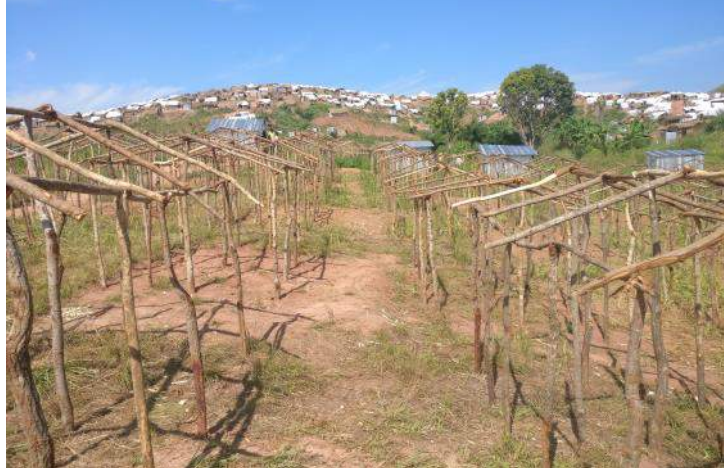
Emergency shelters in Katanika displacement site awaiting tarps and then ready to host IDPs. © IOM 2018 (Photo: IOM Carin Atterby)
