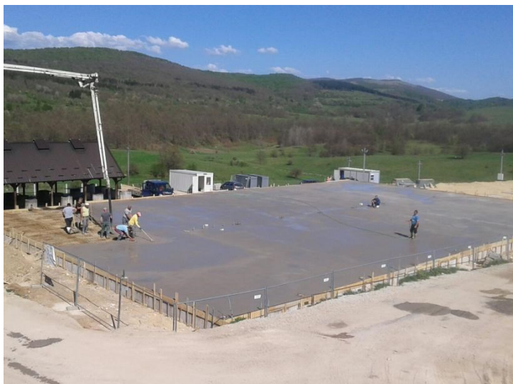
Work on the dining area in TRC Lipa © IOM 2021
