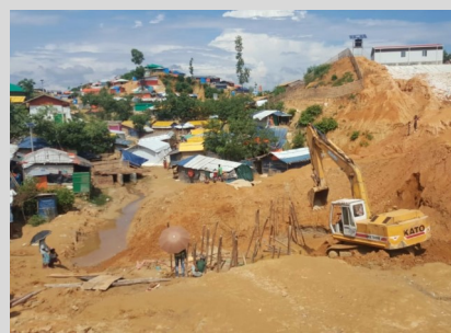
Football Field Road Extension in Camp 10
