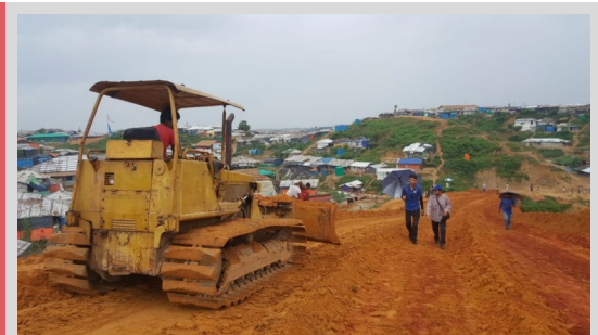
Pan Bazar Road Extension work in Camp 8W.
