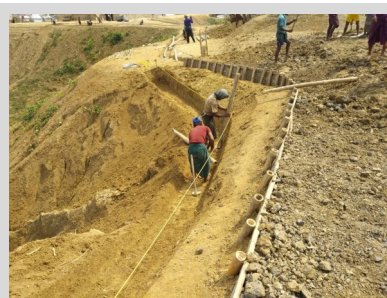
Ongoing stabilization work beside new plots in Camp 20 Extension.
