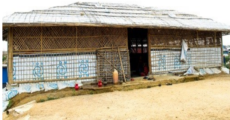
To date, IOM upgraded 58 community shelters, creating temporary shelter space for over 4,419 Rohingya refugees in nine Camps. ©IOM 2018
