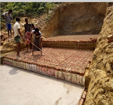
New Desludging tank work ongoing in Camp 18.
