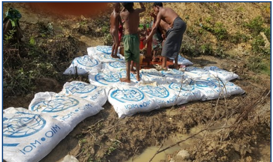
Cash-For-Work activities improve pedestrian access in Balukhali. IOM 2017
