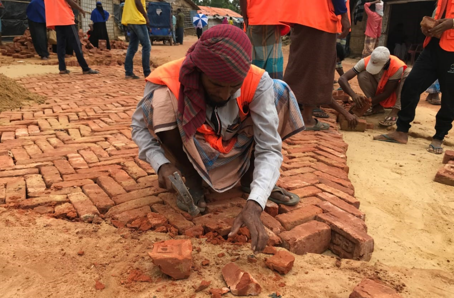
SMEP WORKER SUPPORTS ROAD REPAIR EFFORTS TO ENSURE CAMP ACCESS © IOM 2019
