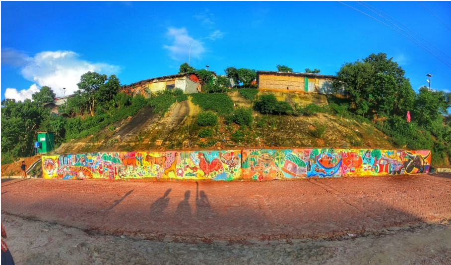
RETAINING WALL IN KBE DEPICTING COLORFUL SCENES FROM LIFE IN THE CAMPS, THANKS TO SMEP COLLABORATION WITH PARTNER ARTOLUTION © IOM 2019
