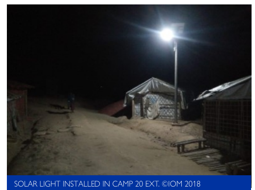
SOLAR LIGHT INSTALLED IN CAMP 20 EXT. ©IOM 2018
