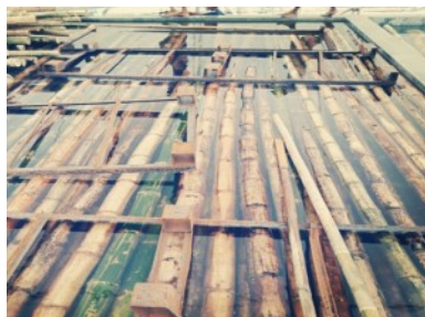
BAMBOO SOAKING IN A WATER-BASED CHEMICAL SOLUTION INSIDE A CONCRETE TANK. © IOM 2018
