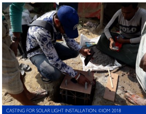
CASTING FOR SOLAR LIGHT INSTALLATION. ©IOM 2018
