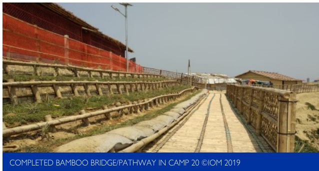
COMPLETED BAMBOO BRIDGE/PATHWAY IN CAMP 20 © IOM 2019
