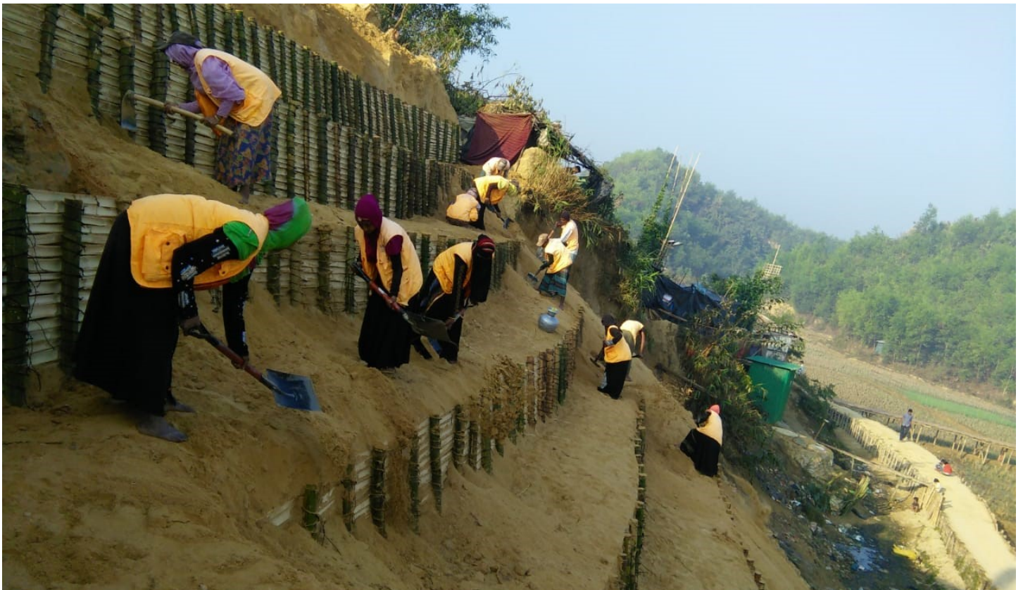
SMEP TEAM STABILISING SLOPES FOR SHELTER RELOCATIONS IN CHAKMARKUL ©IOM 2019.
