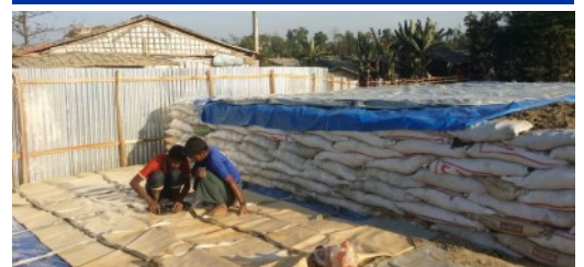
SETTING UP OF BLADDERS FOR WATER SUPPLY IN ALIKHALI (CAMP 25). ©IOM 2019
