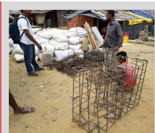
Preparation for installation of lamp posts in Camp 10.
