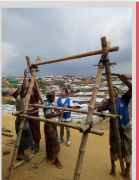
Construction of fire point in Camp 18.
