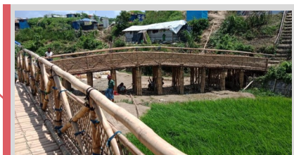
Completed bamboo bridge in Camp 22.
