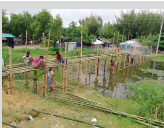
Bamboo bridge construction ongoing in Camp 23.
