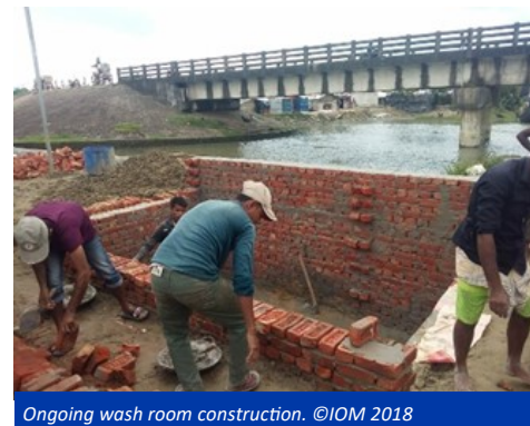
Ongoing wash room construction. ©IOM 2018
