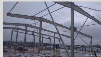
Ongoing assembly of Camp 3 IOM Health facility steel structure ongoing.
