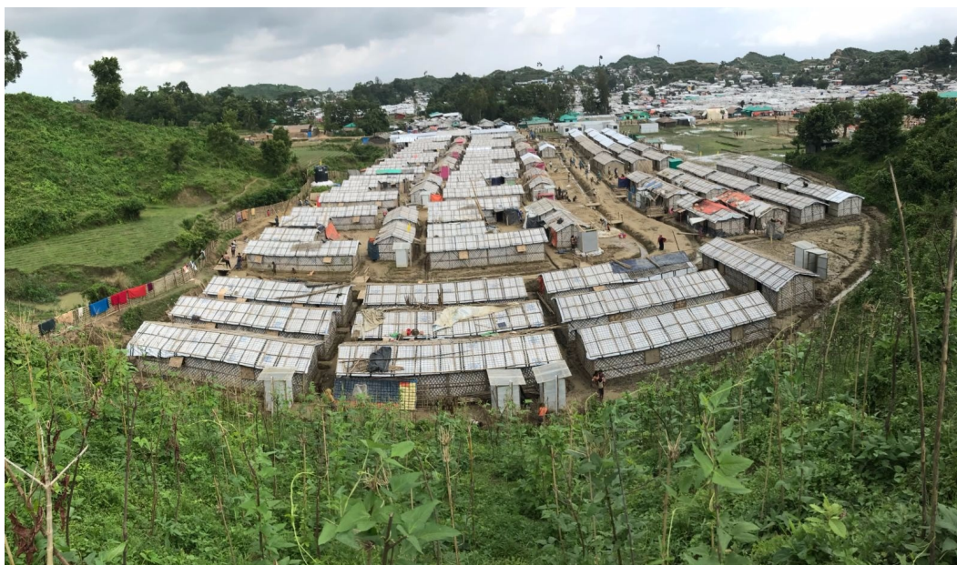
Overview of development in Unchiprang relocation site, with 163 Transitional Shelters. ©IOM 2018
