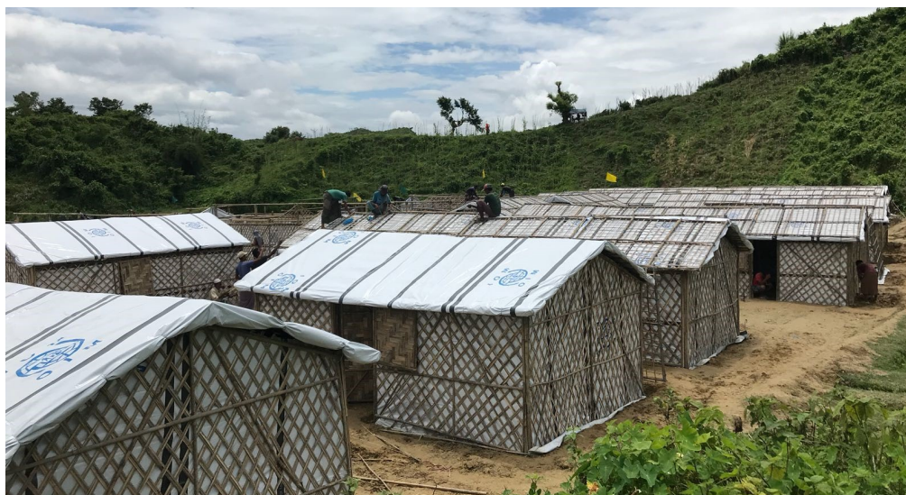
IOM has now constructed 163 robust emergency shelters to relocate the most at-risk families in Unchiprang (Unchiprang, August 2018). ©IOM 2018
