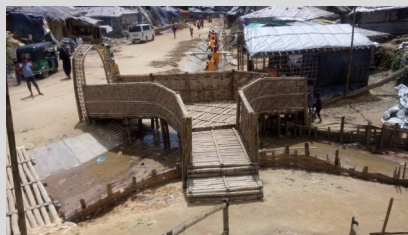
Completed 3-Way Bamboo Bridge in Camp 9.
