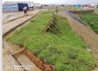
Pathway protection, stabilisation & grassing in Camp 20 Extension.
