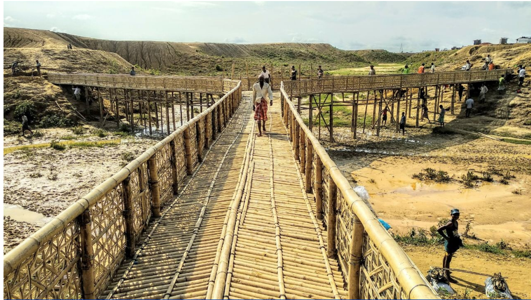
One of the three-way bridges constructed in Camp 20 Extension. ©IOM 2018
