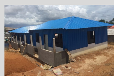
IOM nearly completed the construction of a police post in Camp 1.
