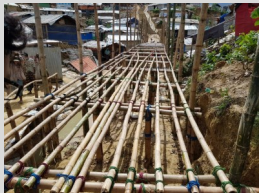
A bridge along a porter route is under construction in Camp 18.
