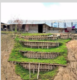
Stabilization work stage 1 in Camp 20 Extension.
