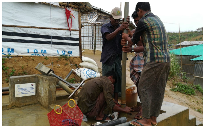
DTW repair in Kutupalong-Balukhali Expansion Site. ©IOM 2018
