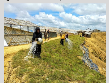
Women involved in CfW watering grass planted for slope stabilisation
