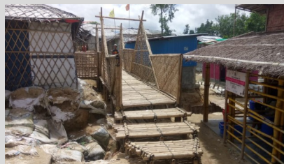
Bamboo bridge and stairs in Camp 9
