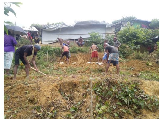
On-going dislodging tank construction in Camp 18.
