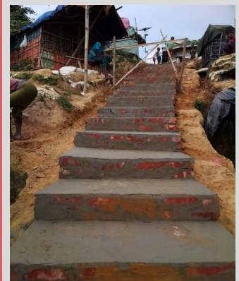
Construction of stairs on a porter route.
