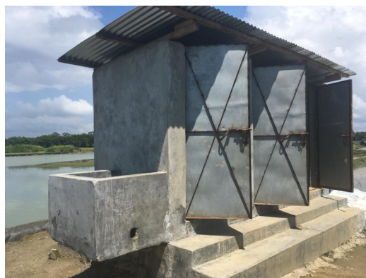
Construction of community latrines in Shamlapur. ©IOM 2018
