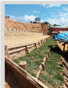
Retaining wall constructed in Camp 18 along Army Road.
