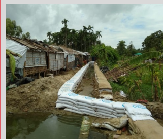
Diversion canal drainage (picture above) as well as main drainage covered by bamboo (picture below) in Purbo Assarbonia, Shamlapur.
