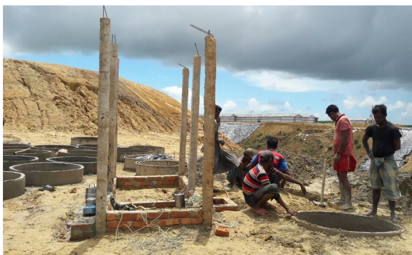
Construction of latrines in Camp 20 Extension.
