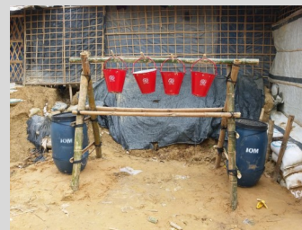
A total of 60 fire buckets have been installed in Camp 10.
