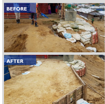
“Before-after” filling and leveling works at the entrance of a school.
