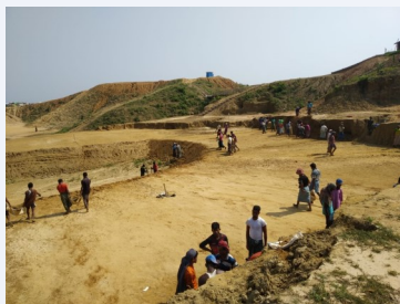
Land preparation to increase habitable area in Camp 20 Extension.
