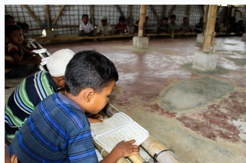
A concrete floor was part of the upgrades. ©IOM 2018
