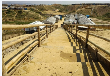
Construction of brick stairs with handrail.
