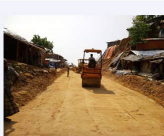
Pan Bazar road construction.
