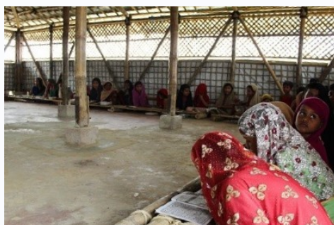
The structures of the Mosque was reinforced. ©IOM 2018
