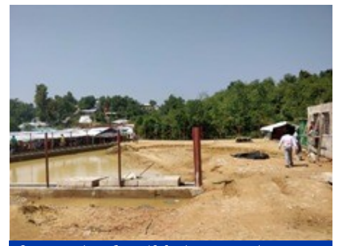
Ongoing works in Camp 12 for the water supply project. ©IOM 2018
