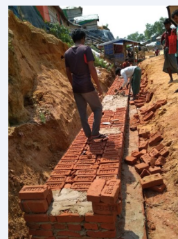
Retaining structures on Pan Bazar road.
