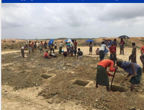
1. Digging holes to place the pillars in the ground
