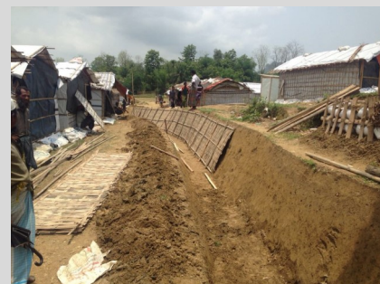
Morover, drainage works are ongoing at the relocation site in Unchiprang.
