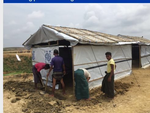
4. Fixing plastic sheeting around the shelters
