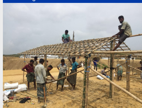
2. Building the structural framework
