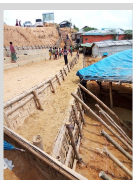
Slope reinforcement along the Army Road in Camp 18.
