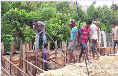
Boundary wall casting in Camp 12.
