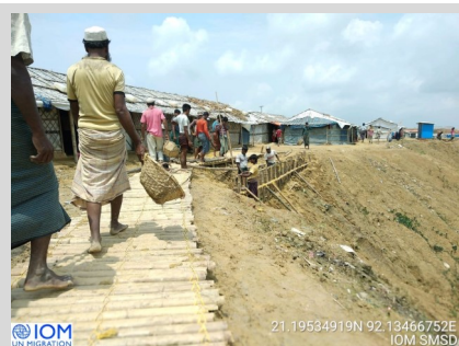
Stabilization work and bamboo pathway in Camp 20 Extension.
