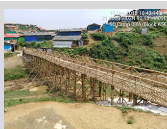
Completed bamboo bridge in Camp 8W.
