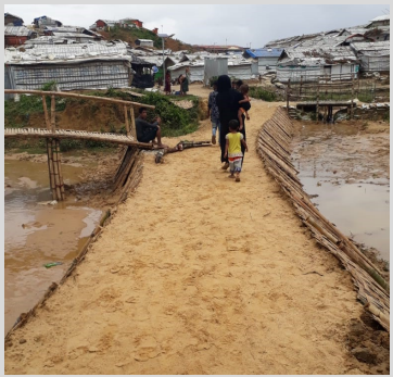
New path, slope protection and bridge.
