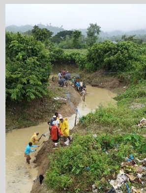
Excavation and removing silt from the canal in Unchprang
