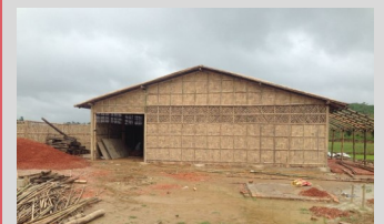
Construction of a storage/tools warehouse is almost completed in Unchprang.
