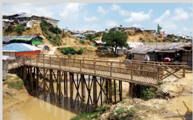
Bridge constructed between Camp 12 and 18.
