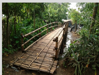
Newly completed bamboo bridge at Possim Assarbonia - Shamlapur.
