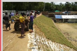
Slope stabilization with grass planting.
