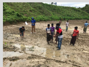
Land preparation for the relocation of households at risk of landslides.
