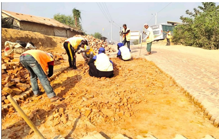
SMEP WORKER SUPPORTS ROAD REPAIR EFFORTS TO ENSURE CAMP ACCESS © IOM 2019
