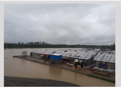
In Hatkhula Para Mitigation camp, the level of water went high before low tide. The areas, that had been backfilled as a preparedness measure, did not get flooded despite heavy rains and the high tide.
