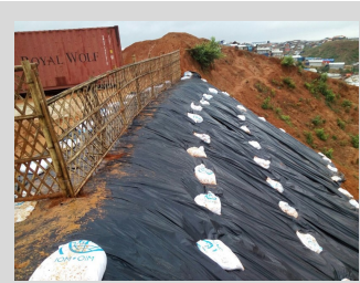
Protecting earth embankment in Camp 10.
