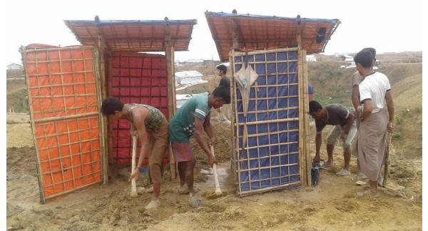
Repairs of damaged latrines in Camp 20 extension. ©IOM 2018
