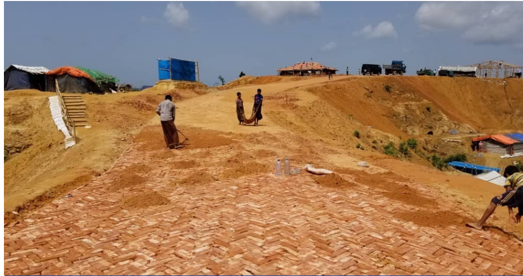
Construction of Football Field Road extension. ©IOM 2018
