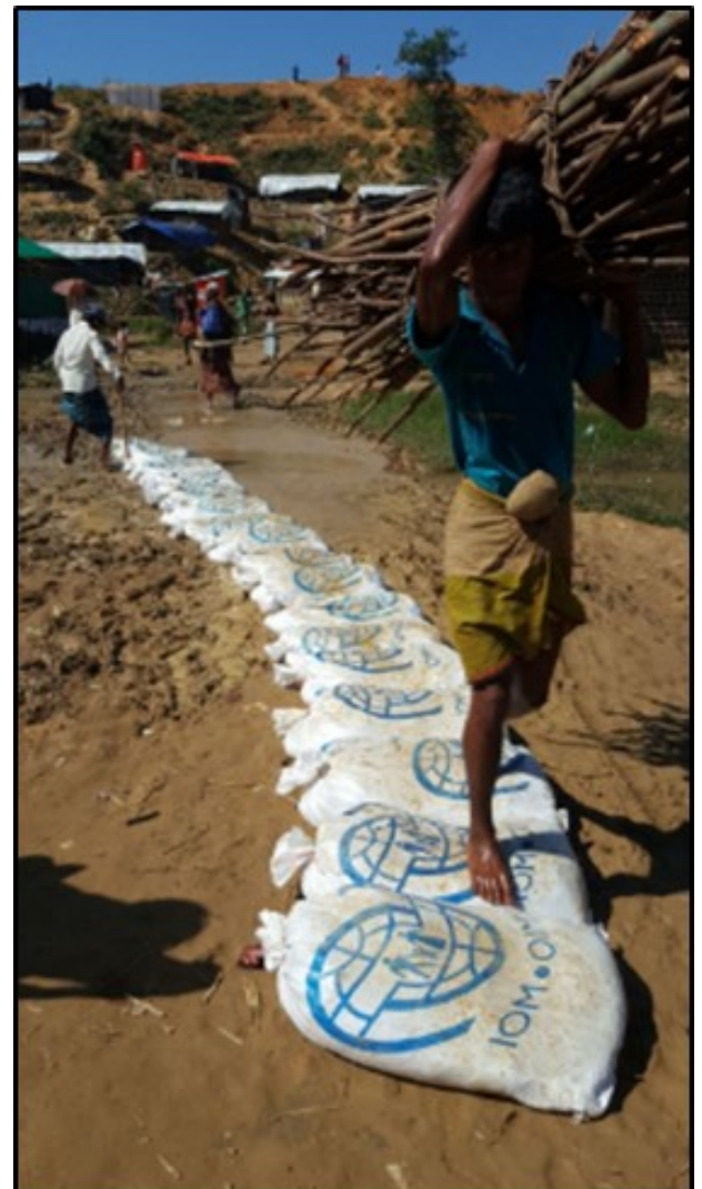
Site improvements and levelling works for communal service facilities. IOM 2017
