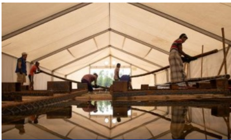
BAMBOO BECOMES INSECT-RESISTANT WHEN SOAKED IN A CHEMICAL SOLUTION FOR 12 -14 DAYS. © IOM 2018/ABDULLAH MASHRIF
